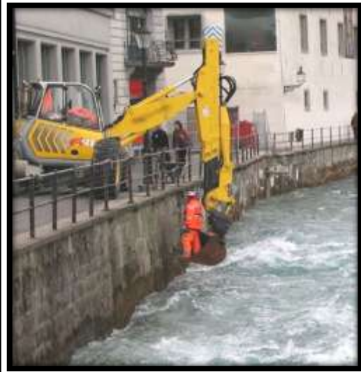
excavator ≠ proper scaffold
